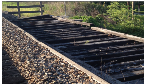
Peavine trestle bridge over NC 226
