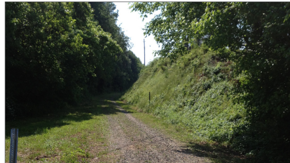
City-owned Peavine Rail Corridor
