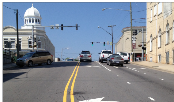
Steep grades are present on Court Street, headed east to Main Street
