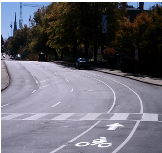
Bike lanes on Salisbury Street in Raleigh, NC were installed during a resurfacing project.
